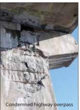
Modern concrete, without pozzolan, is almost always a disaster waiting to happen. It is just a matter or time before unconverted CH degrades the concrete.
